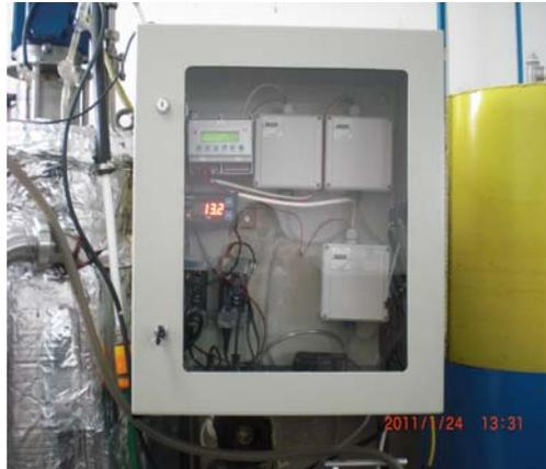
Fig. 7 Sensors for CH<sub>4</sub>, CO<sub>2</sub> and H<sub>2</sub> into the biogas
