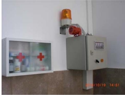
Fig. 12 Light and sound signalling of the protection system
