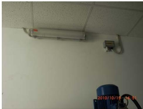
Fig. 13 Light signalling of the protection system
